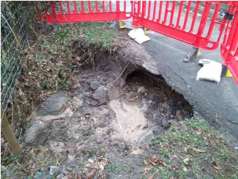
Effects of excess run-off: Soils Erosion (Image: LLong)
